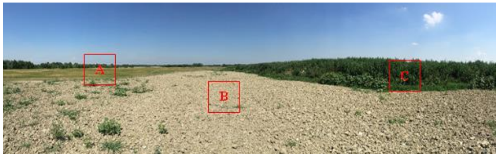
Figure 2. Closed landfill: [A] human transported material; [B] reconstituted soil; [C] natural vegetation on reconstituted soil.
